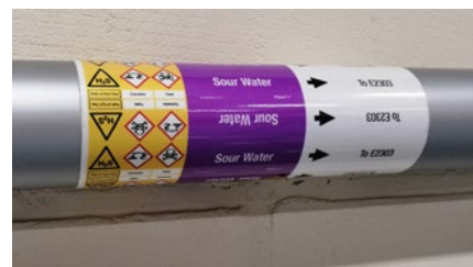
Pipe Marking according ISO 20560-1
